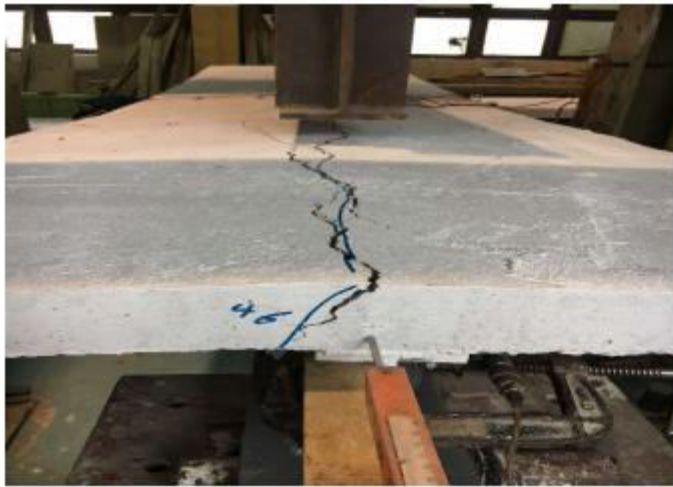
(a) Longitudinal cracks
