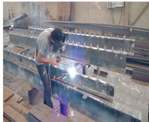
(a) Welding of shear connectors
