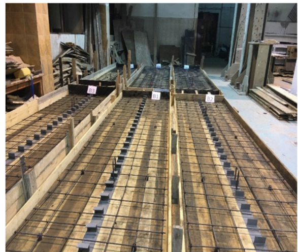
(b) Formwork and reinforcement mesh
