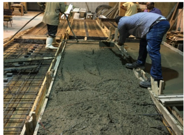
(c) Concrete pouring.
